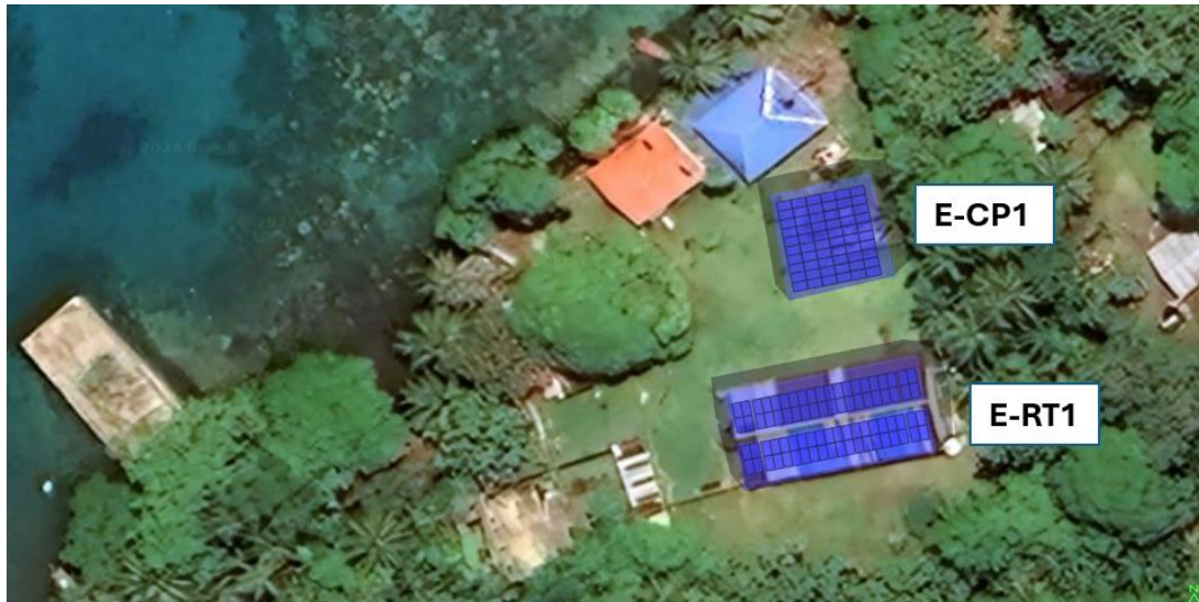
Figure 28. Top view of PV arrays in Etten
