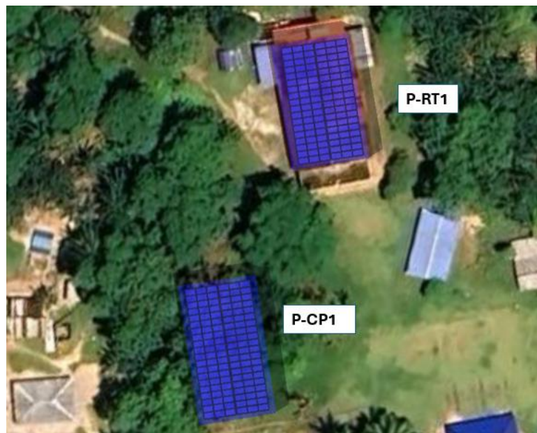
Figure 30. Top view of PV arrays in Piis Paneu
