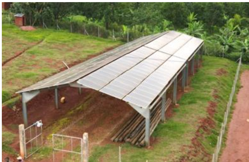
Figure 27. Example of a 3 m high canopy installation (waterproofed for Etten and Piis Paneu). Source: TTA
