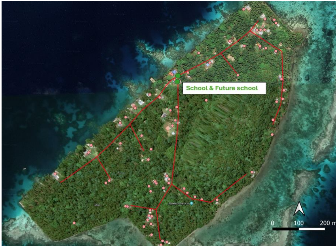
Figure 22. The two PV installations in Etten island
