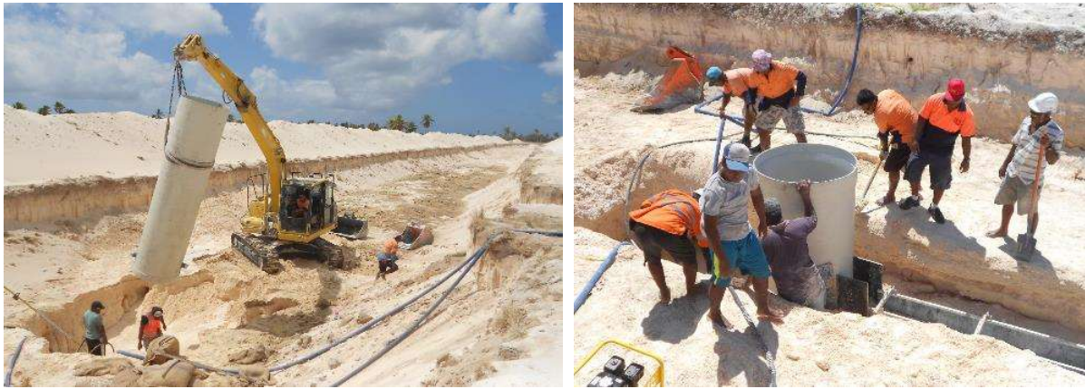
Figure 17. Gallery construction at the Decca lens during the IDWSKIP project
