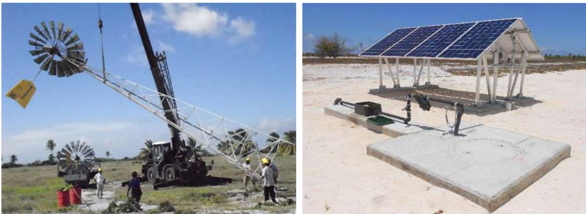
Figure 18. Wind pump rehabilitation (left) and new solar pump (right)
