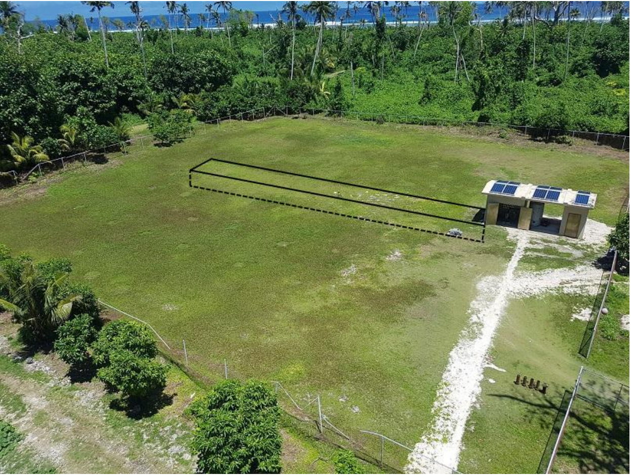
View of groundwater catchment area and pumphouse. The sketch indicates the trench that was dug for the two horizontal wells (pipes) to be installed. The trench was then refilled with sands.
