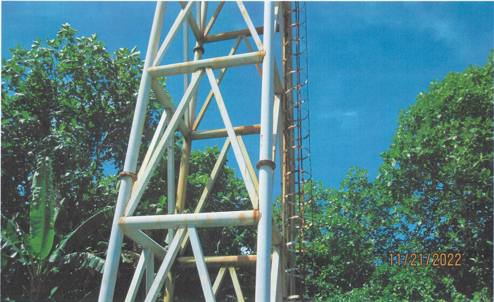
Existing ladder leading up to existing 5,000 U.S Gallon capacity water tank
