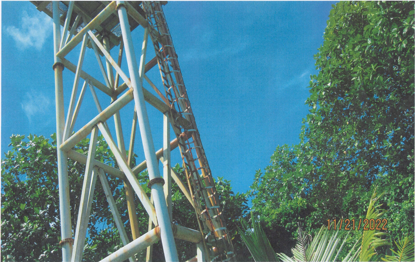
Existing ladder leading up to existing 5,000 U.S Gallon capacity water tank
