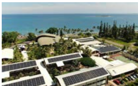
A total of 1200 m 2 of solar panels will help save about 455 tonnes of CO 2 per year
