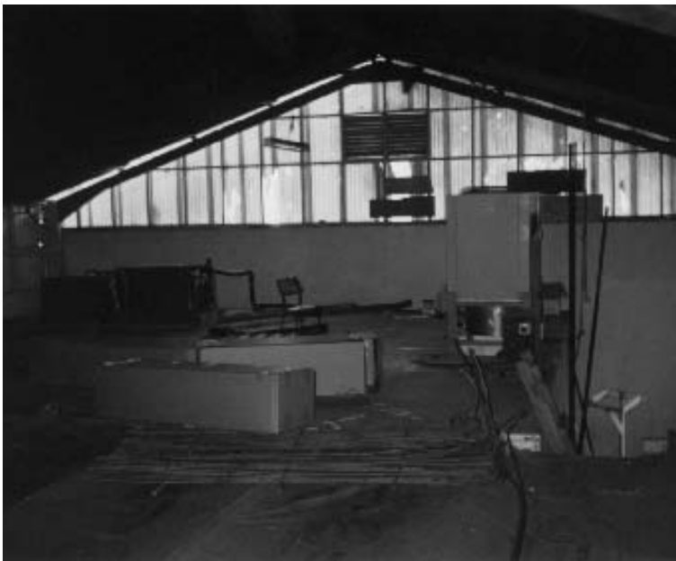
Figure 21: Ice machine mounted inside building over chill room
