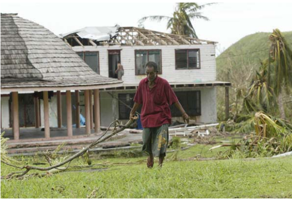
The Samoan fale remained intact whilst the European house took a beating in Fitiuta, Ta'u, American Samoa in the wake of Cyclone Olaf (Photo: Barry Markowitz)
