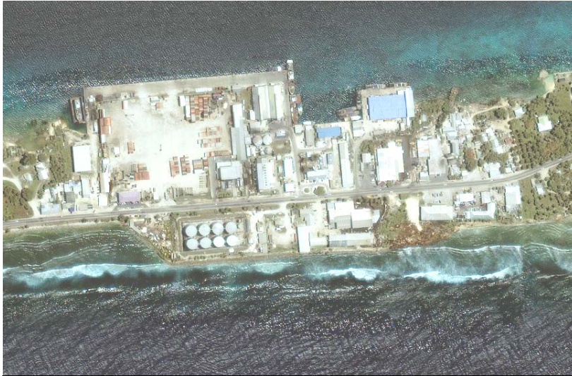
MEC Power Stations and Tank Farm near the Delap dock on Majuro
