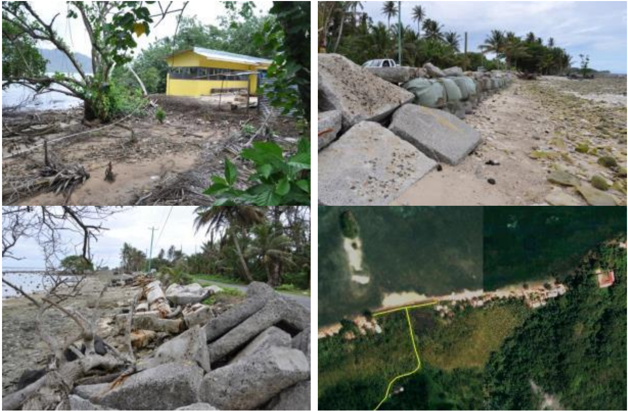
Figure 1-5: Recent examples of poor development activities that will lead to further coastal hazard-related problems and are not sustainable or effective in the long-term. Top left: Low-lying reclamation for a new laundromat at Tafuyat, Lelu Harbour; Top right: Concrete bag seawall to protect the road at Mosral, Malem; Bottom left: Dumped concrete rubble to attempt to protect the road at Pal, Malem; Bottom right: Access road construction through the mangrove and along the foreshore at Leap, Walung.
