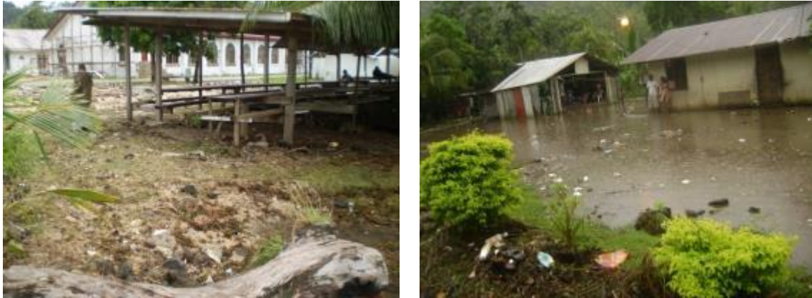
Figure C-3: Debris from overwashing of the seawall at Tafunsak (left) and at Malsu (right) during the swell event of 8-9 December 2008.
