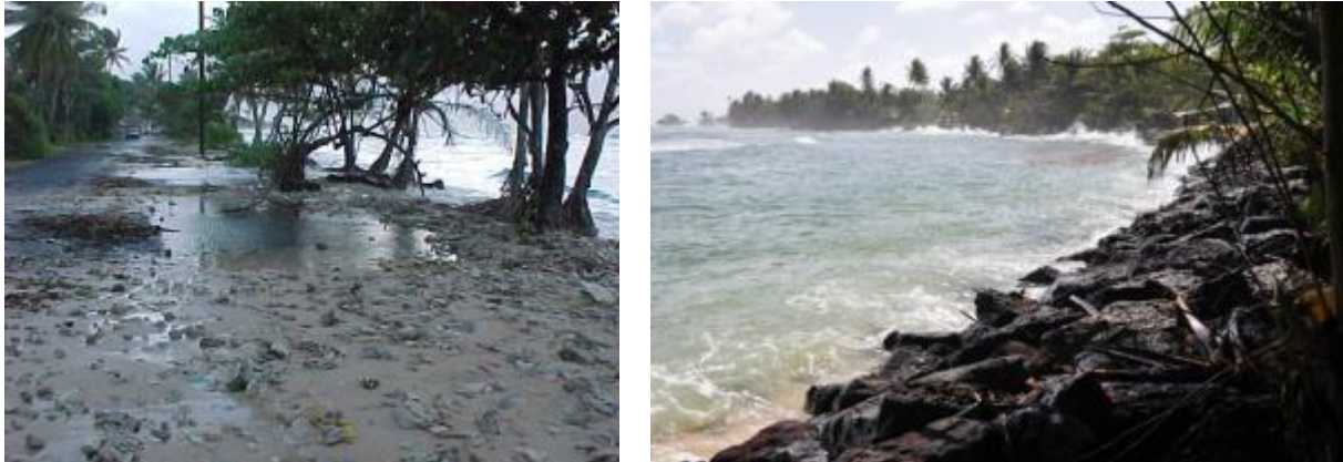
Figure C-2: Wave overwashing at Fukrin in Malem during February 2000 (left) and high tide wave overtopping of the seawall at Malem village during December 2010).
