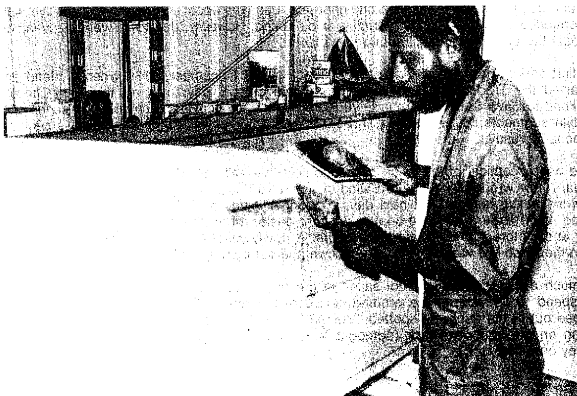
Figure 4: Filling the seams
