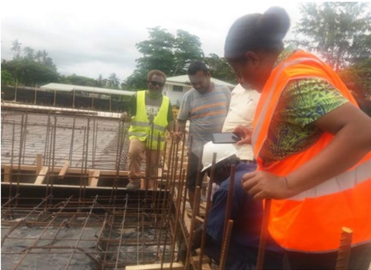
Figure 5. Women inspecting and verifying construction of steel rod bars of the fish ponds. © Nina Lean T. Harry
