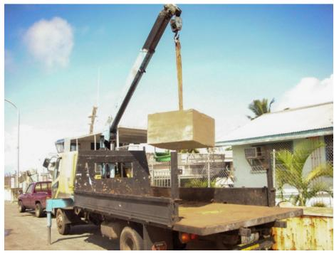
Image 2. Large cement block anchor being lifted by crane for deployment.
