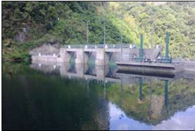
Nadarivatu hydro dam, Fiji
