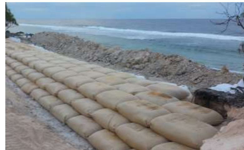
Repairing breach ocean side geotextile bags Funafuti
