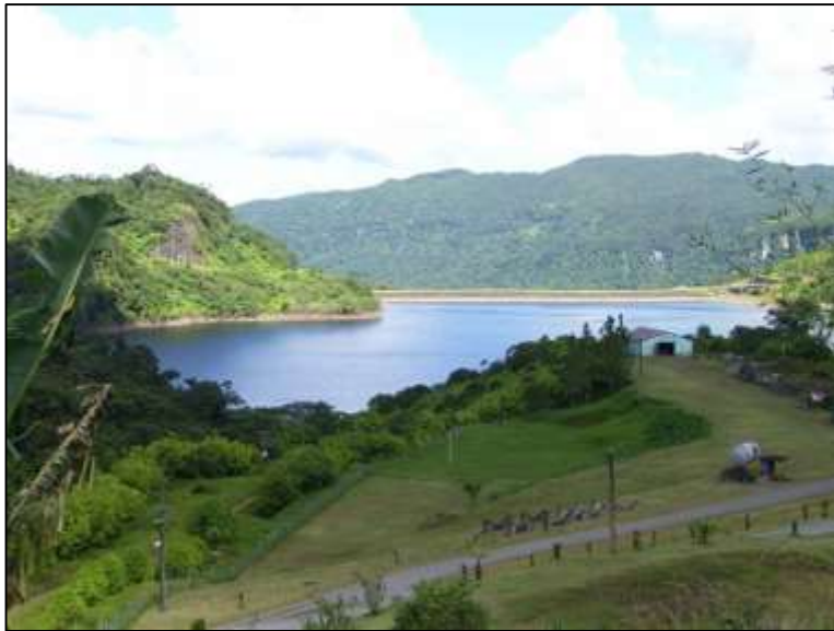
Monasavu Dam, Fiji: 133,000,000 kL
