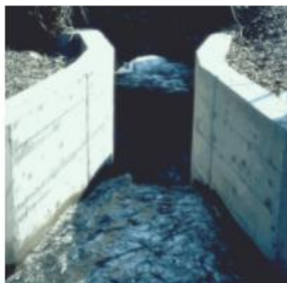
Figure 9 Section contracté / effet venturi, source (12)
