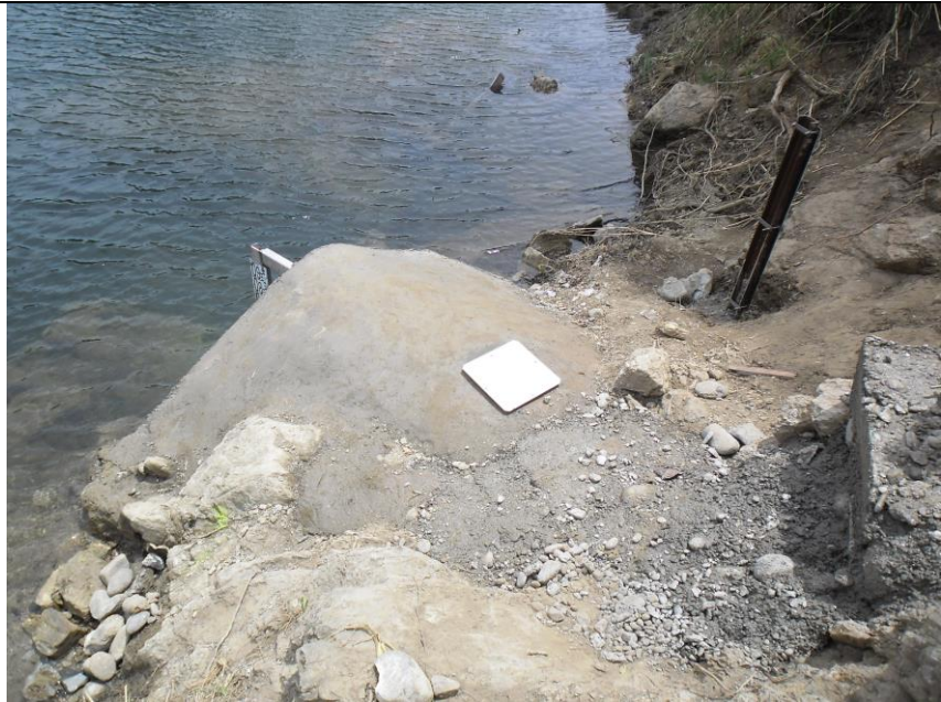
Figure 18 Massif béton terminé, source DAVAR
