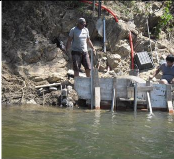
Figure 16 Coffrage et coulage, source DAVAR
